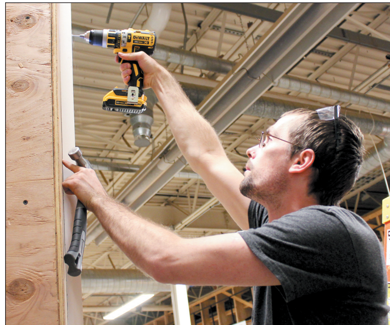
Sean McGinley secures trim around a door inside Middle Bucks Institute of Technology's construction lab.
